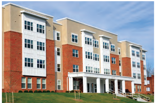
Senior housing constructed by Bon Secours Baltimore. Photo: Bon Secours.
